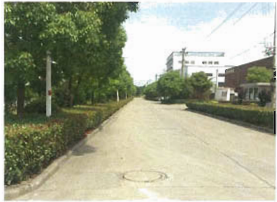
Road on the southern side – Xida Road
