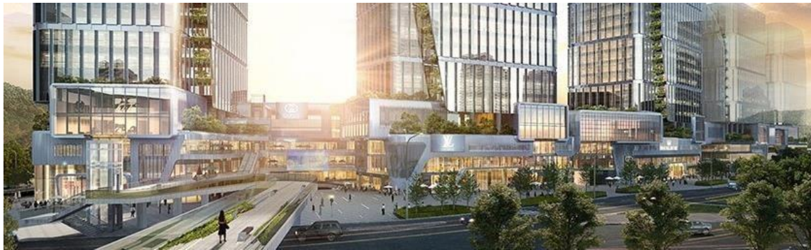
Nam Tai Technology Center Construction of main structure to be completed in 2022
